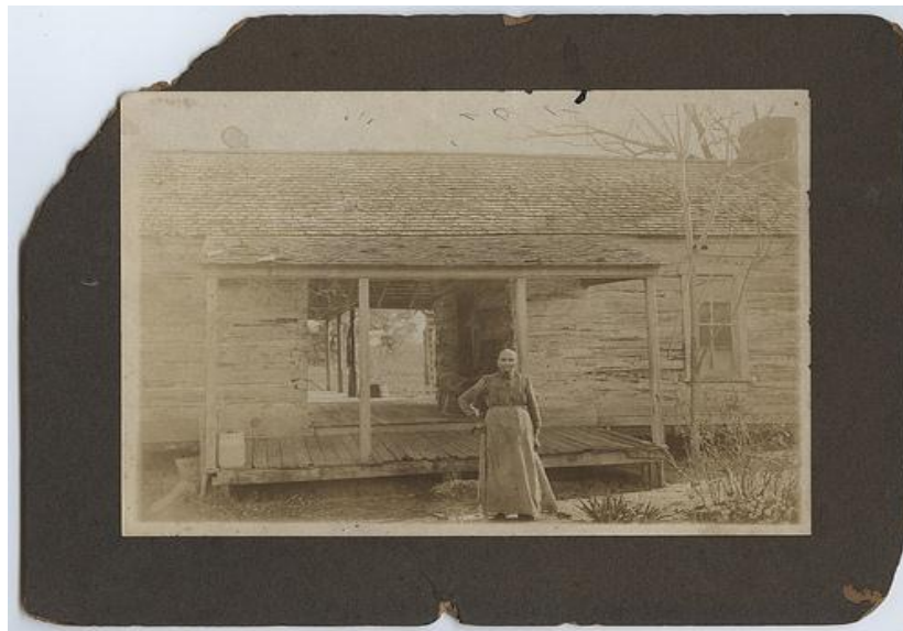
Figure 20: Old Texan "Dog Run" House Log Cabin in Llano County, Texas; source: www.flickrriver.com
